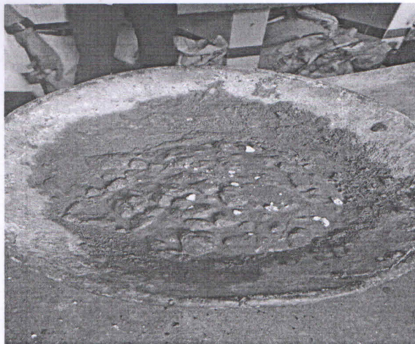
Concrete mixed with chemical waste
